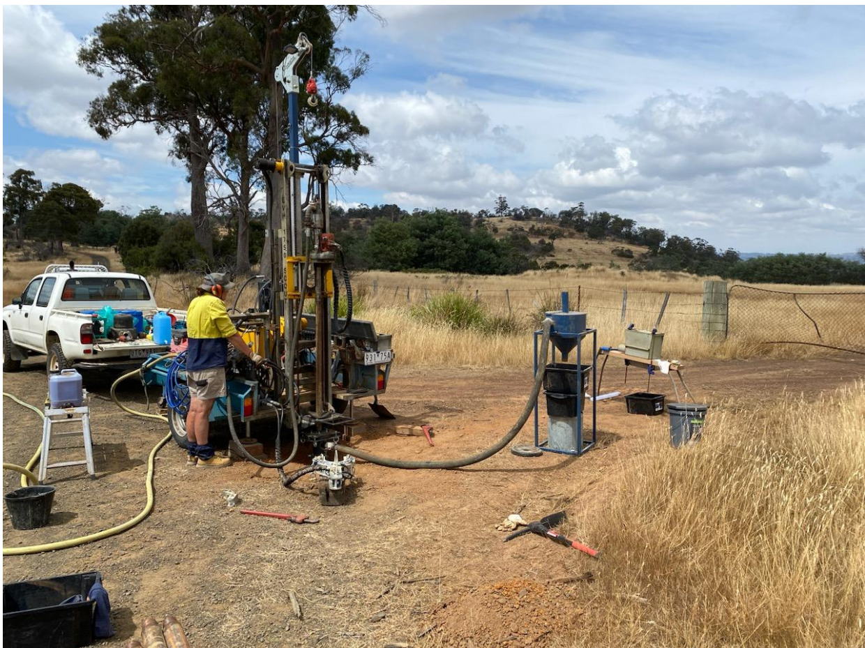
Figure 1: Trailer-mounted drilling rig in use at Russell’s Plains.
